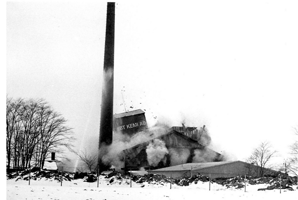
Demolition of the factory, Febr. 22, 1979
